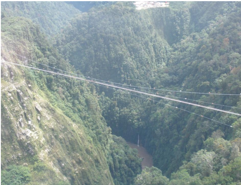
Some spectacular PNG infrastructure. An oil pipeline 500m above the valley floor and 500m across.
