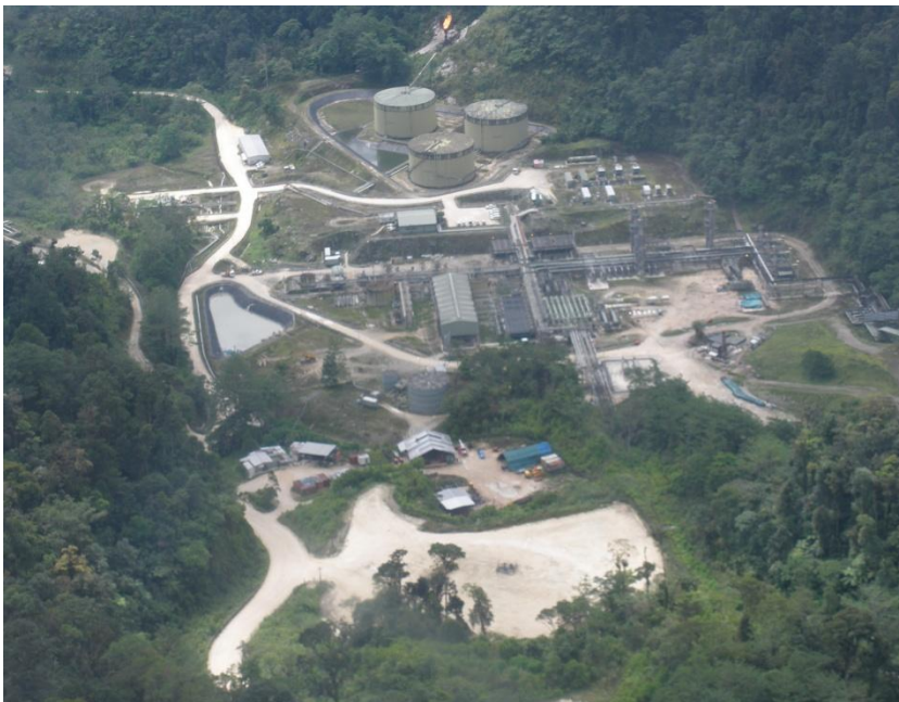
Existing Gas Processing facilities
